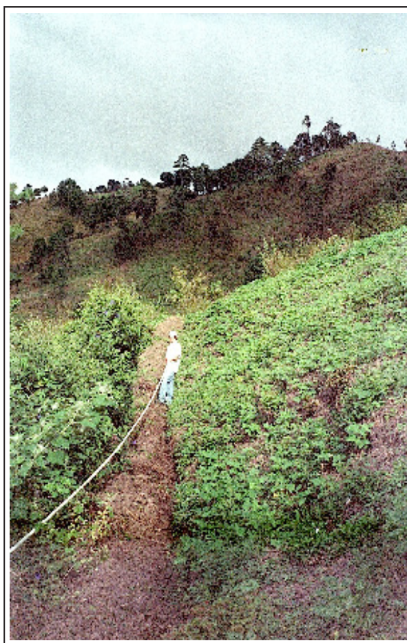
Brian Camblin pulling pipe
